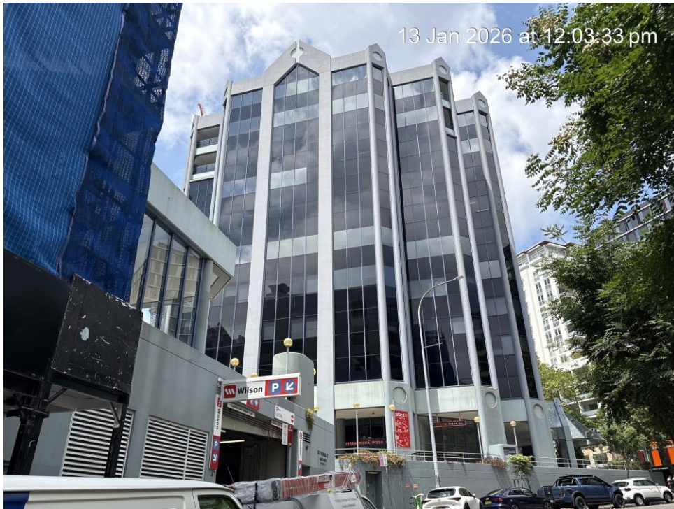
Figure 1: 187-189 Thomas Street, Haymarket viewed from the north-west
